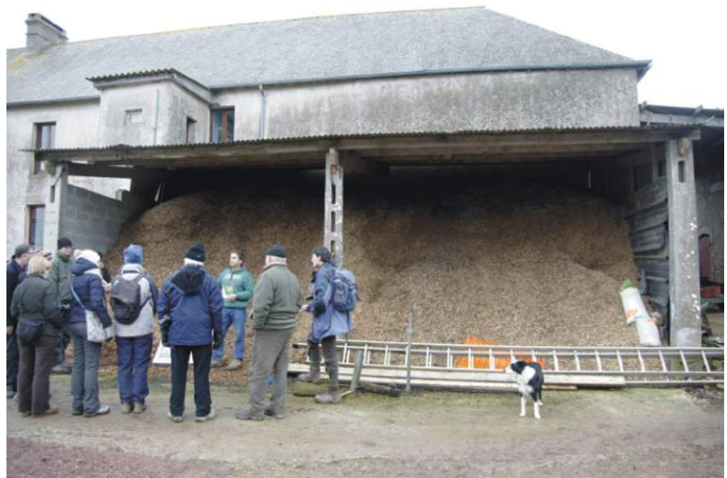
Woodchip drying shed and store at the back of a farmhouse heated with woodchips from farm hedges. The chips self-dry through fermentation. La Tournerie, Raids, Normandy, February 2012.
