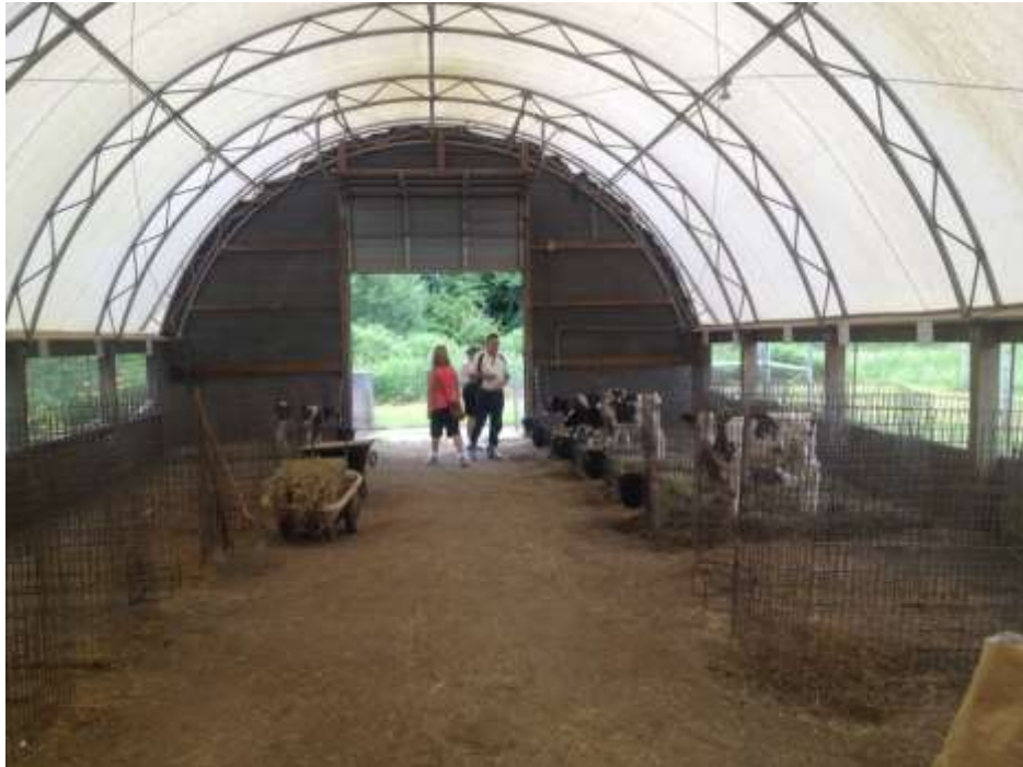
Figure 9: Youngstock accommodation partially funded by the WAC to prevent run off and rainwater contamination from what was previously an open yard
